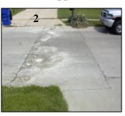
the crack extends the entire width of the street. One can also see that the whole slab has been replaced at one time. This, of course, is evidence of more serious movement problems. There is no rigid type material that will hold these two, separately moving pieces together. The problem has to be addressed below the slab.
