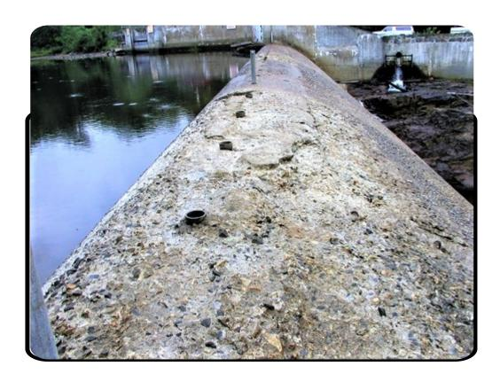
Much of the area had erosion as deep as 6" and breaking away. It was filled in one lift and feather-edged on the sides.
